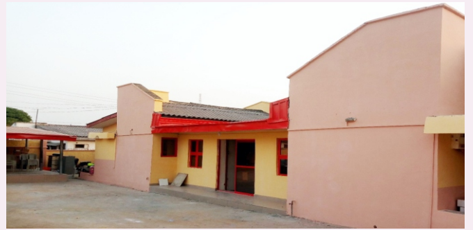
NEW KOGI OFFICE
