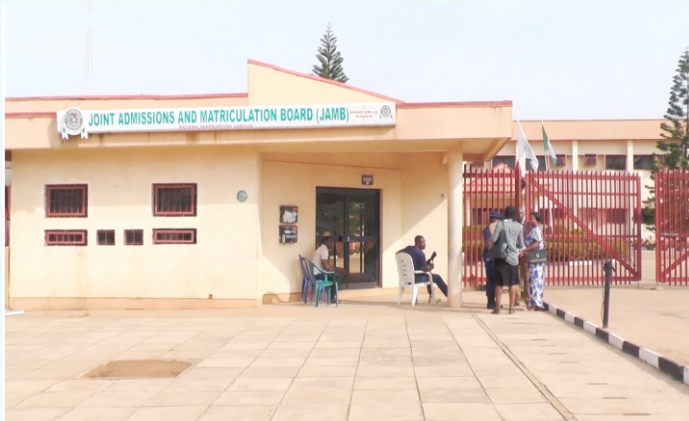
OLD GATE HOUSE AT THE HEADQUARTERS
