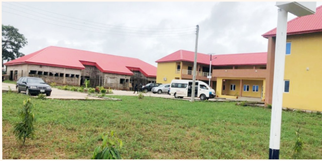
NEW BENIN OFFICE AND ONGOING MEGA CBT CENTRE
